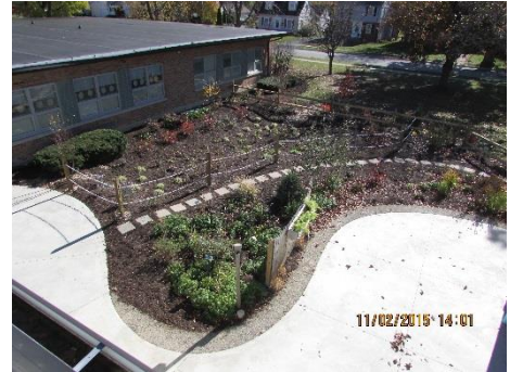
Picture of pervious pavement around rain garden at Jefferson Primary School in Findlay.
